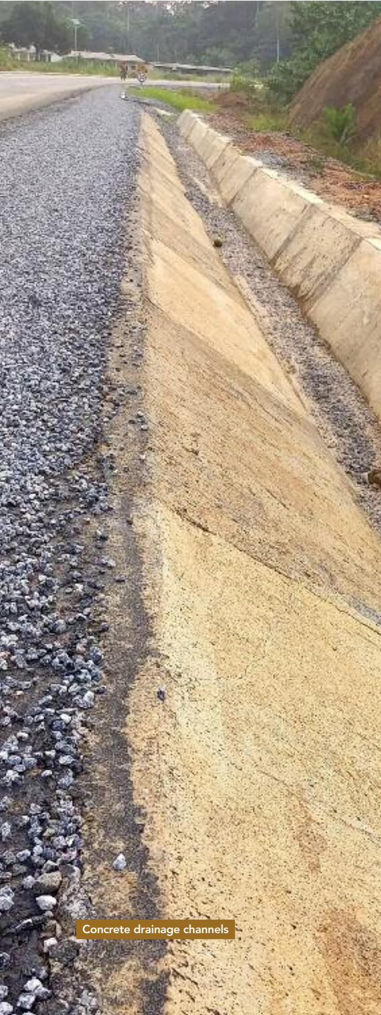
Concrete drainage channels
