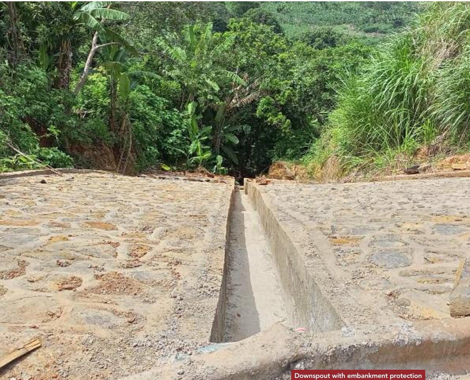
Downspout with embankment protection
