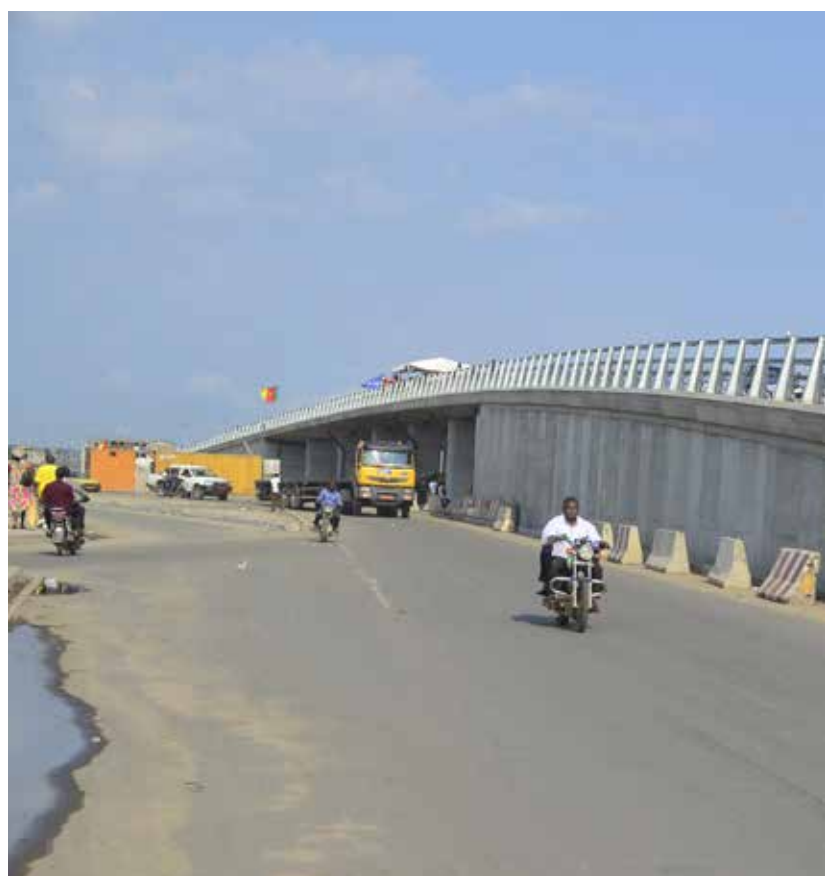
Overpass – Eastern entrance of Douala
